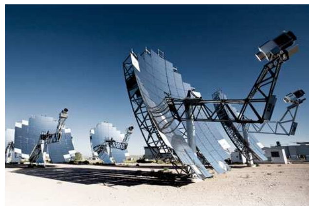
Figure 4 Grouping of planar mirrors into a parabolic shape
