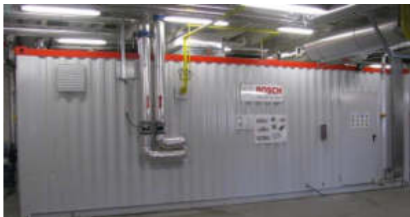
Figure 5 Container with cogeneration unit
